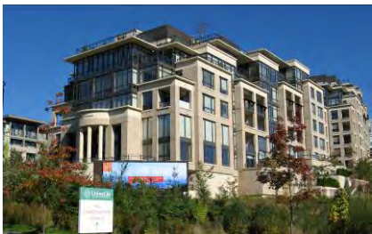
Terraced mid-rise buildings
