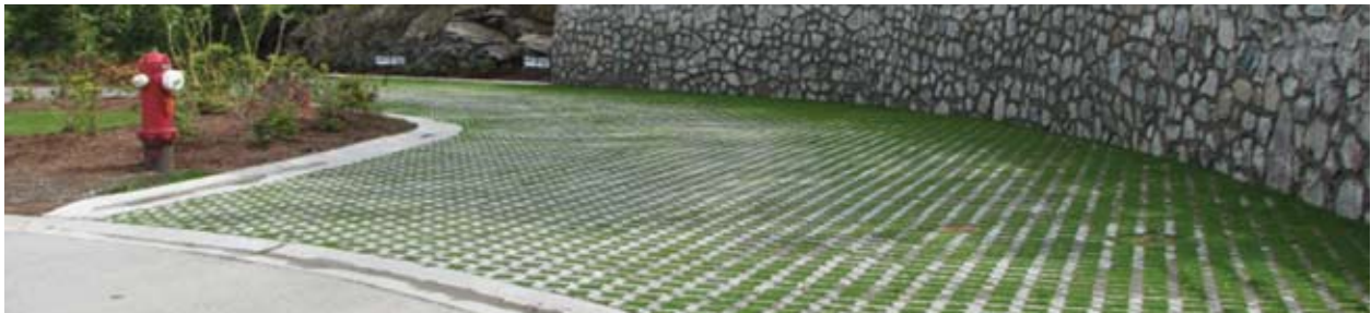
Stormwater Management ~ South Wilkinson Valley
