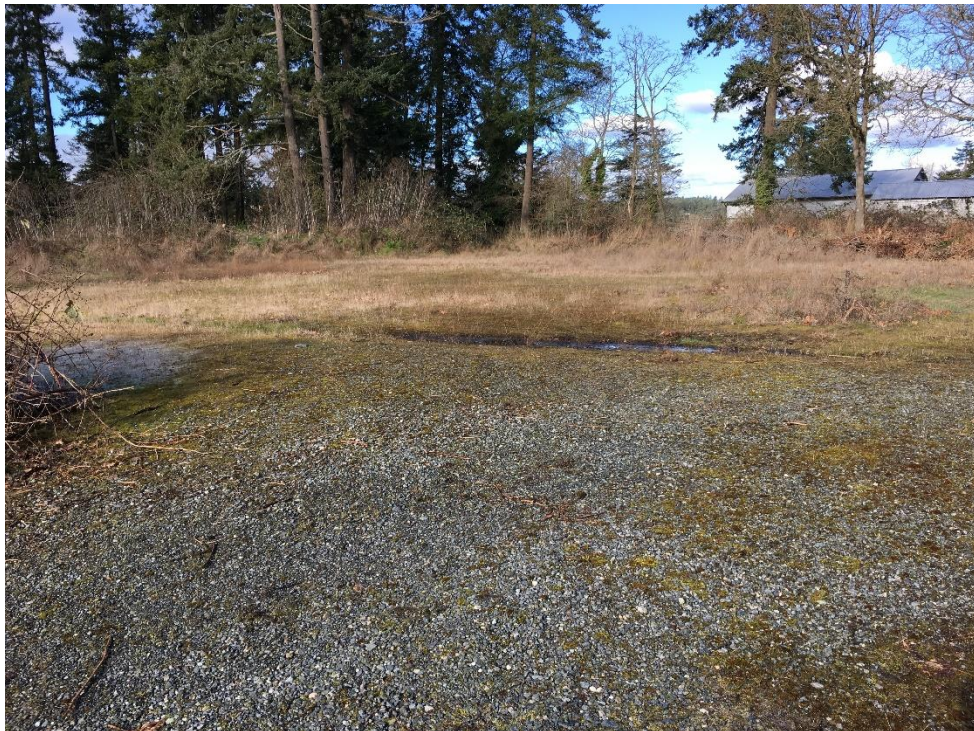
Photograph No.26: Road grade fill placed in the central northern portion of the Site adjacent to the former plant nursery and in the area where soil segregation formerly occurred
