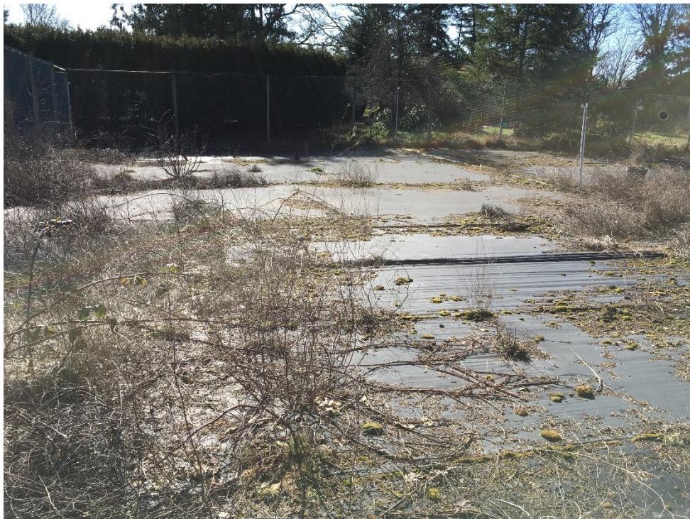
Photograph No.10: Geosynthetic fabric lining the ground surface of the former plant nursery
