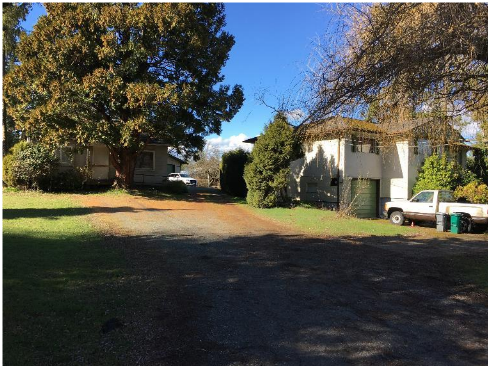
Photograph No.4: View west of 1447 Burnside Rd W (left side of photo) and 1449 Burnside Rd W (right side)
