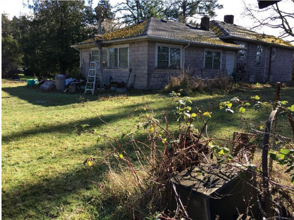
Photograph No.7: View northwest of house on southwest corner of the Site at #5 Helmcken Rd
