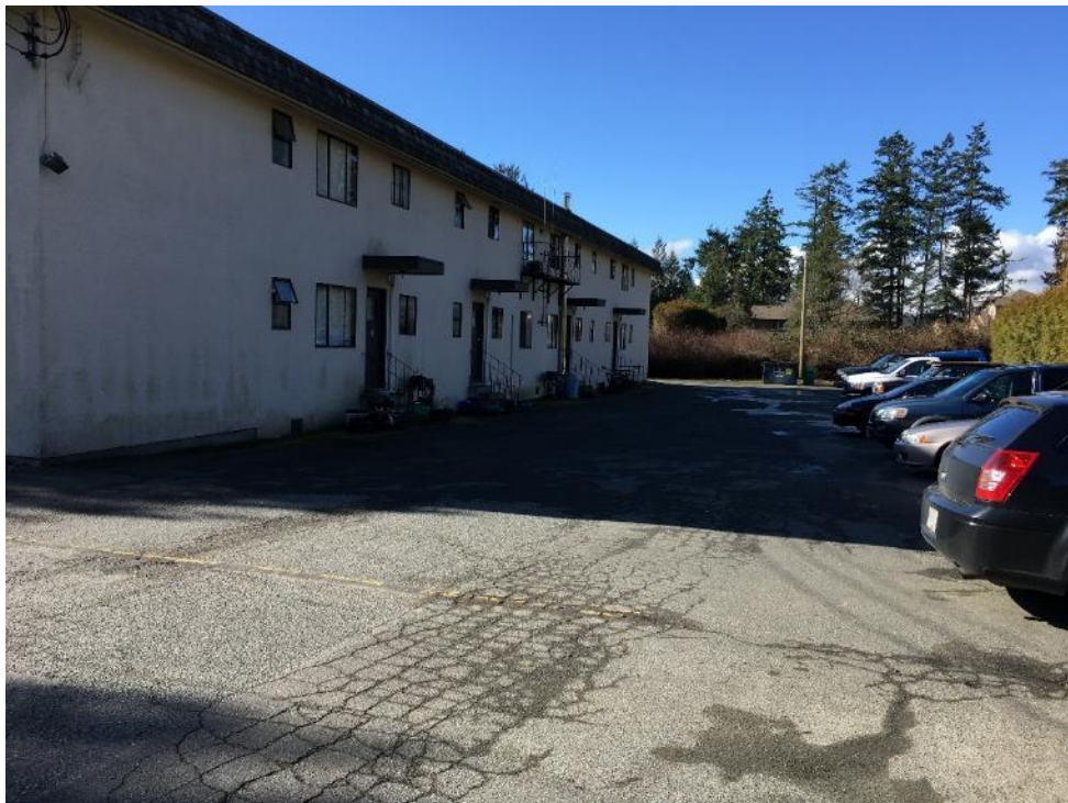
Photograph No.2: The parking lot on the north side of the Robalee Apartment Building at #3 Helmcken Rd.
