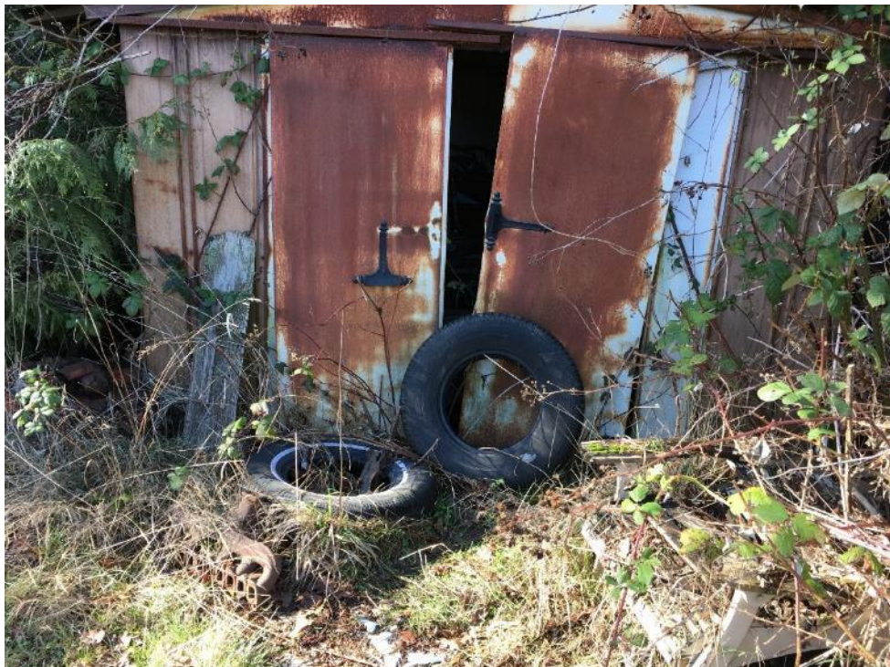
Photograph No.8: Detached garage/shed along the western boundary of the Site for # 5 Helmcken Rd
