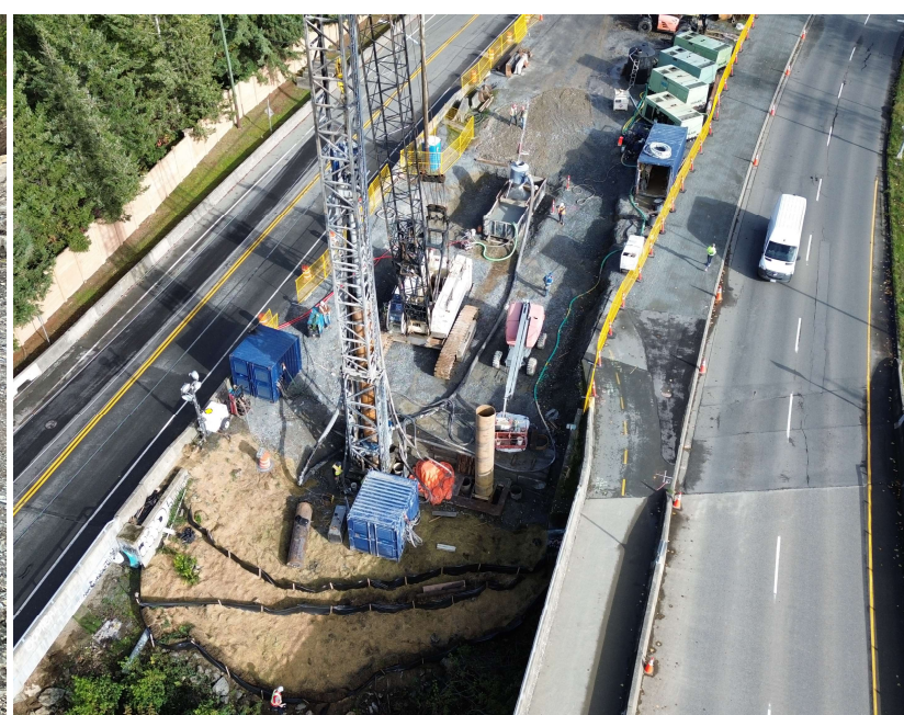
Pile installation for GGT multi-use bridge
