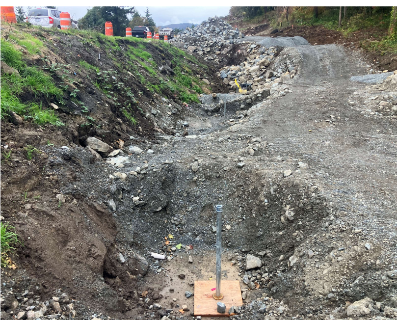
Embankment fills and installation of settlement gauges near Wilkinson Lift Station
