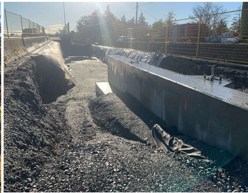
Portage Road retaining wall construction
