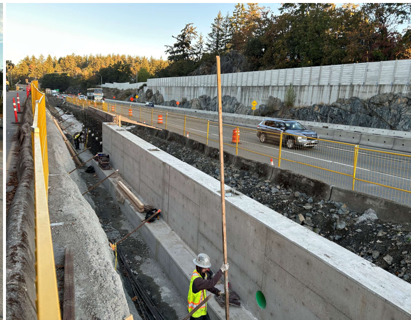
Portage Road retaining wall construction
