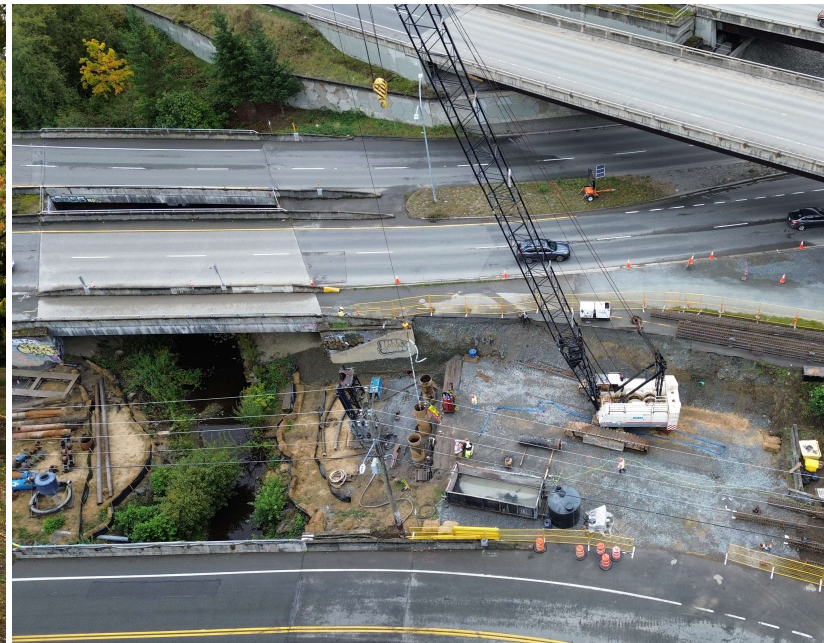
Pile installation for GGT multi-use bridge
