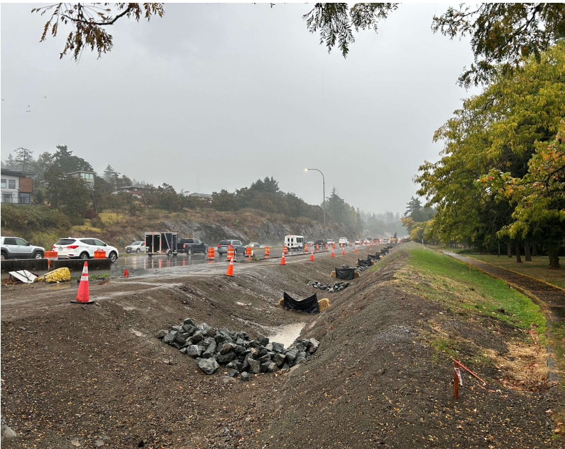
Drainage works along Highway 1 (southbound) near Portage Linear Park
