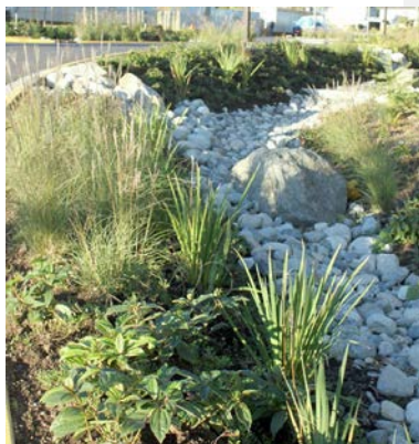
Bioswale. Source: Capital Regional District.
