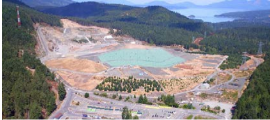
Hartland Road Landfill. Source: Capital Regional District.
