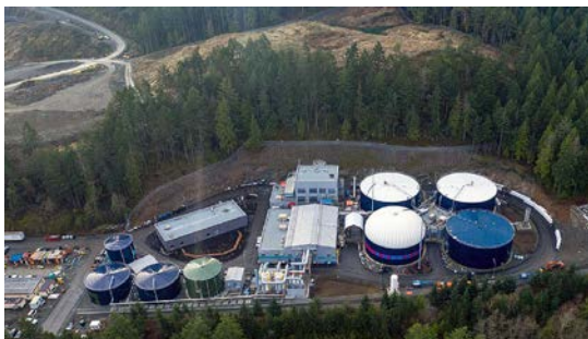
CRD Wastewater Treatment Plant. Source: Victoria News.
