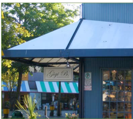
Awnings provide weather protection for sidewalks.
