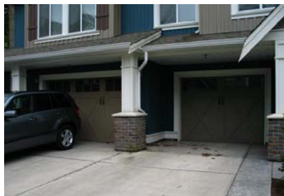
Tandem parking and shared driveways, with the garage inset to reduce the size and appearance.
