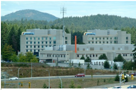
Image 19 Victoria General Hospital Source: C. Marshall
