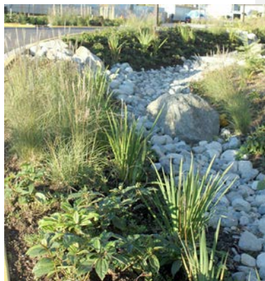
Bioswale. Source: Capital Regional District.
