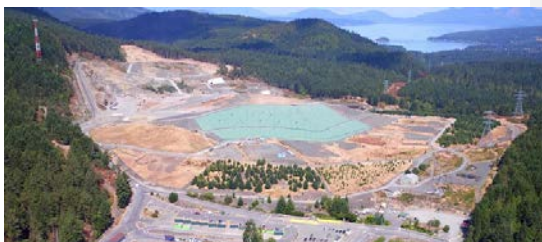
Hartland Road Landfill. Source: Capital Regional District.
