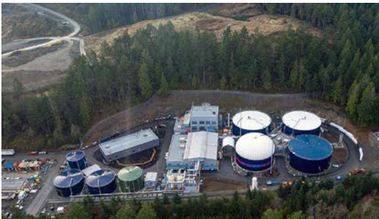
CRD Wastewater Treatment Plant. Source: Victoria News.
